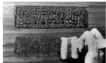
Fig. 38: Priming by brush
